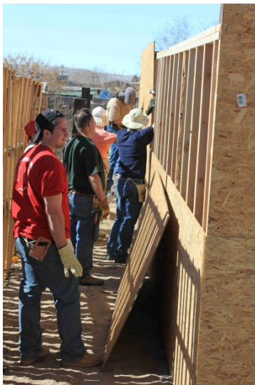
Adding the sheathing
